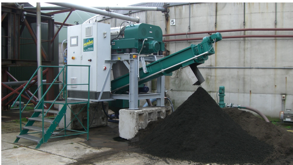
Plug & Play - sludge dewatering unit with CT-450 decanter centrifuge - location Germany
